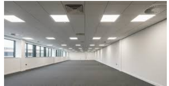
Commercial Lighting Repairs
