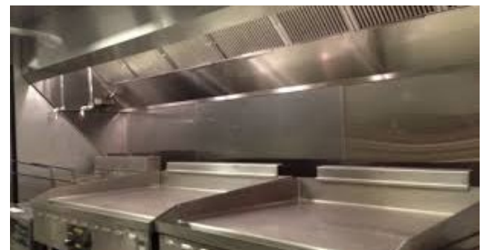
Hood and Exhaust Cleaning
